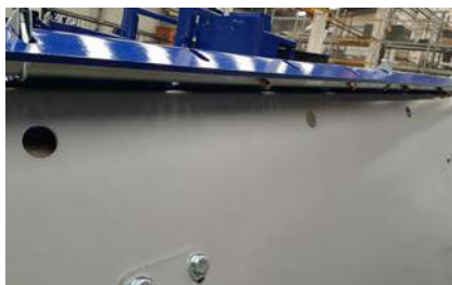
Dust Suppression System and Water Pump
